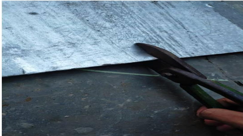
Rajah 3.8 Memotong plat besi
